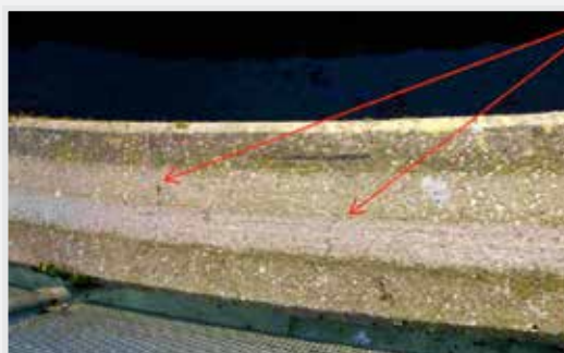
Some surface cracking at intervals otherwise track is relatively smooth.
