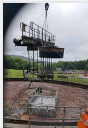
Removal of PST bridge by crane.
